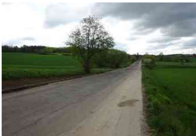
Sanace krajnice v km 9,500
