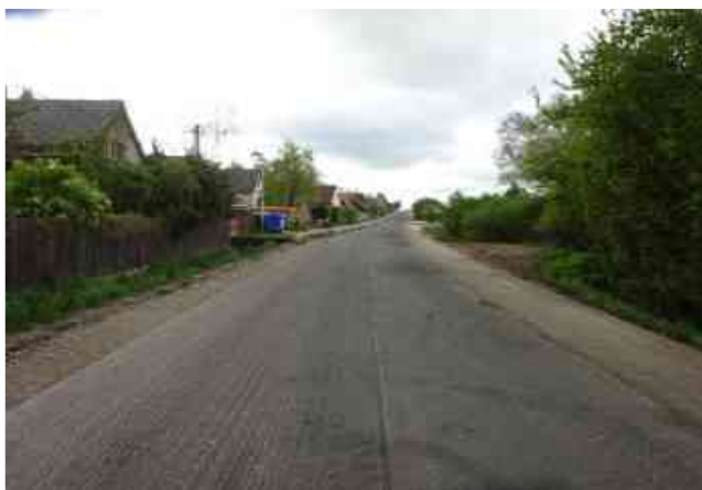
Sanace krajnice v km 10,000
