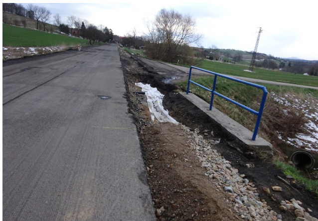
Sanace krajnice v km 9,600
