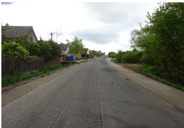
Sanace krajnice v km 10,000
