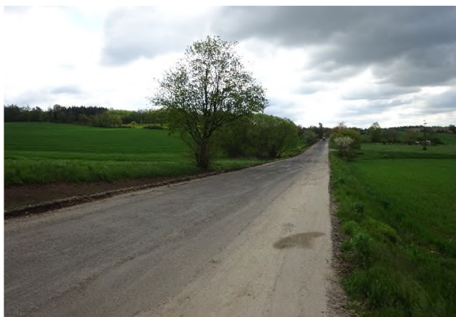
Sanace krajnice v km 9,500
