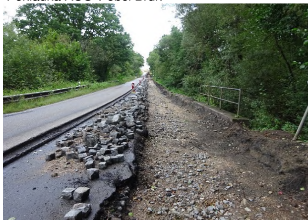
Sanace krajnice v KM KM 13,320-14,260
