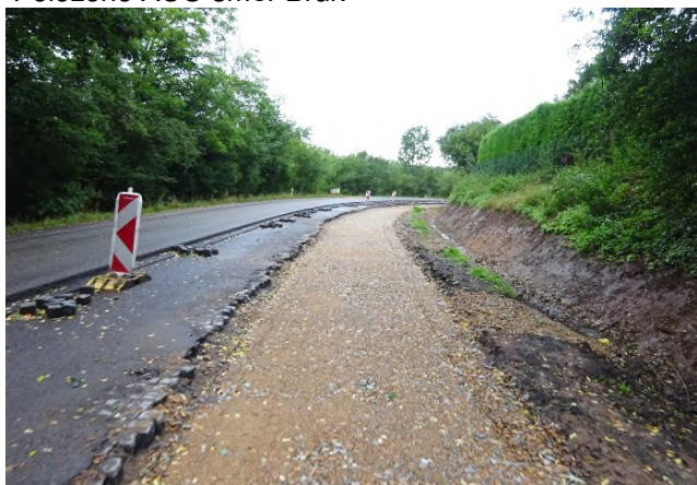
Sanace krajnice v KM KM 13,320-14,260
