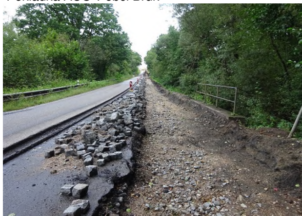
Sanace krajnice v KM KM 13,320-14,260
