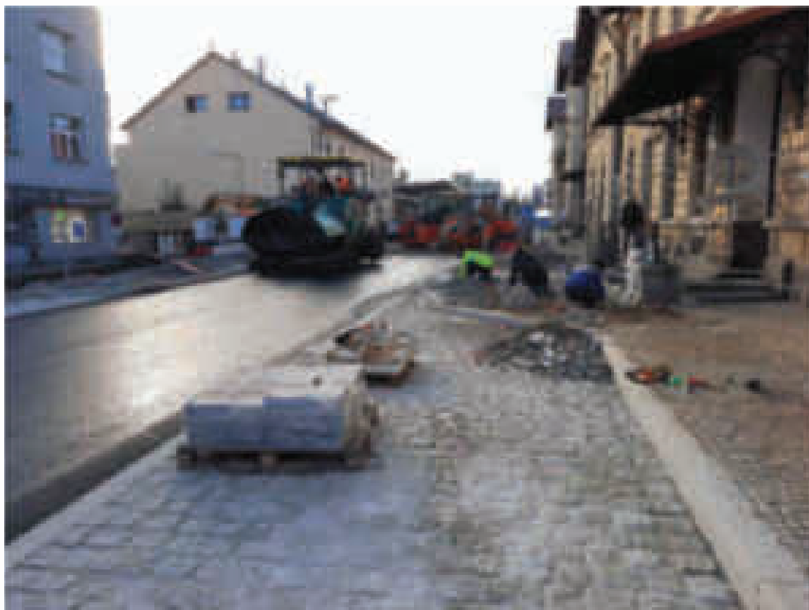
Figure 1. Street construction site.
