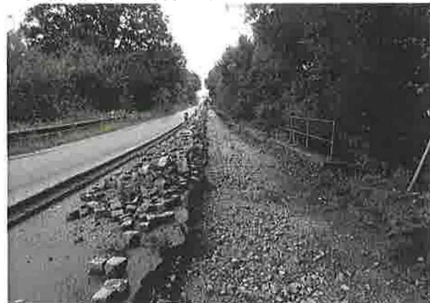
Sanace krajnice v KM KM 13,320-14,260
