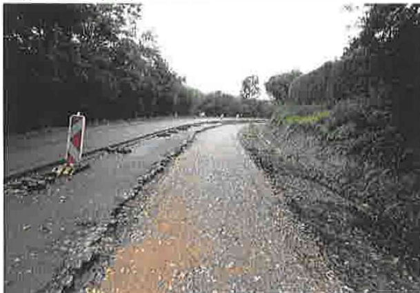
Sanace krajnice v KM KM 13,320-14,260
