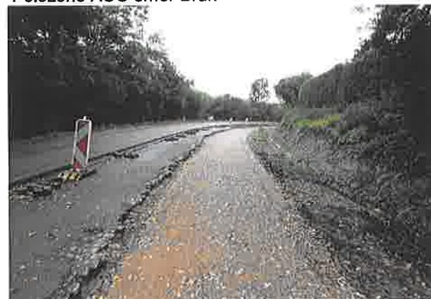
Sanace krajnice v KM KM 13,320-14,260
