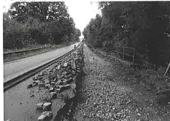
Sanace krajnice v KM KM 13,320-14,260
