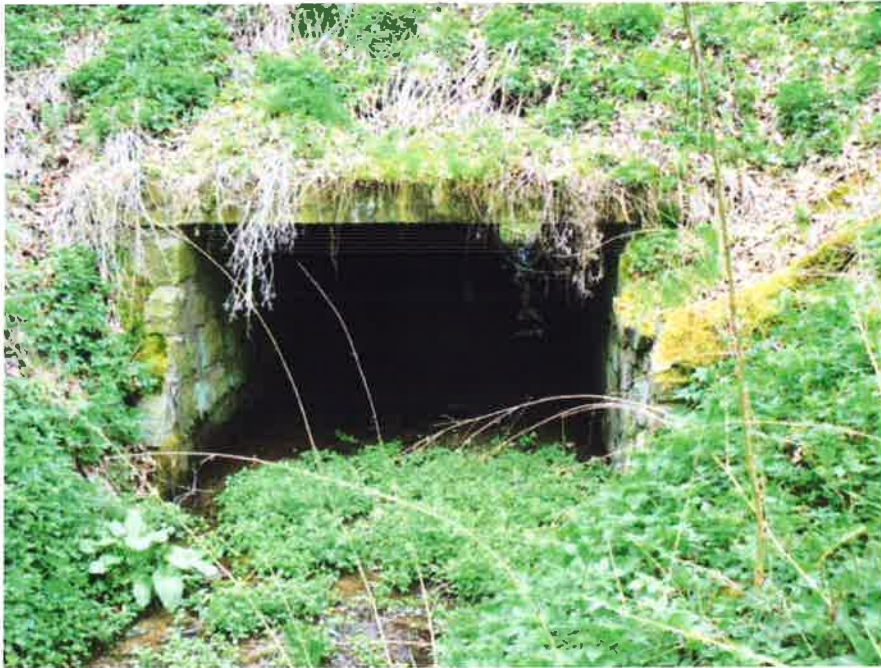
II/105, most ev.č. 105-020
