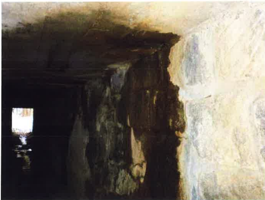
II/105, most ev.č. 105-020
