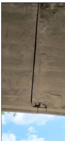
Ozub 4 - detail spáry
